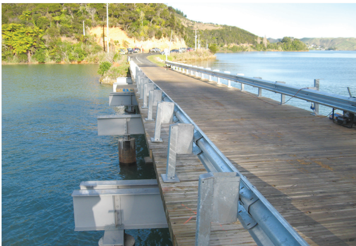
Harbour Road Bridge, Te Waitere
