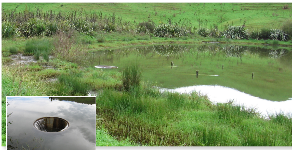
Stormwater drain, Walker Road
